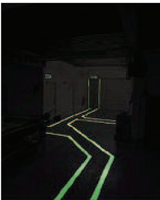
Figure 49: A 'way-guidance' system
