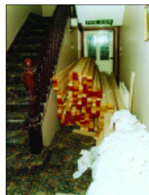
Figure 9: A blocked corridor with incorrect signage
